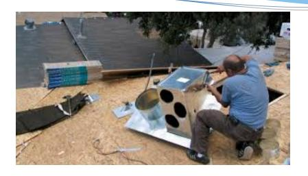
At 9:20 a.m. on January 5, 2018, an employee was installing HVAC unit ducts. The employee fell from a roof opening onto a concrete floor and was killed due to head trauma.
